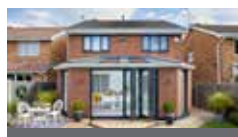
New Build Warm Rooms
