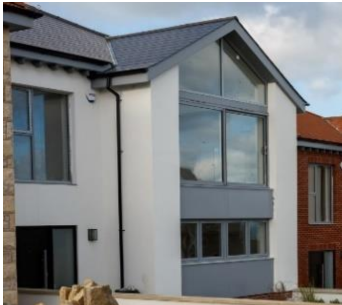
Fascias, soffits and guttering
