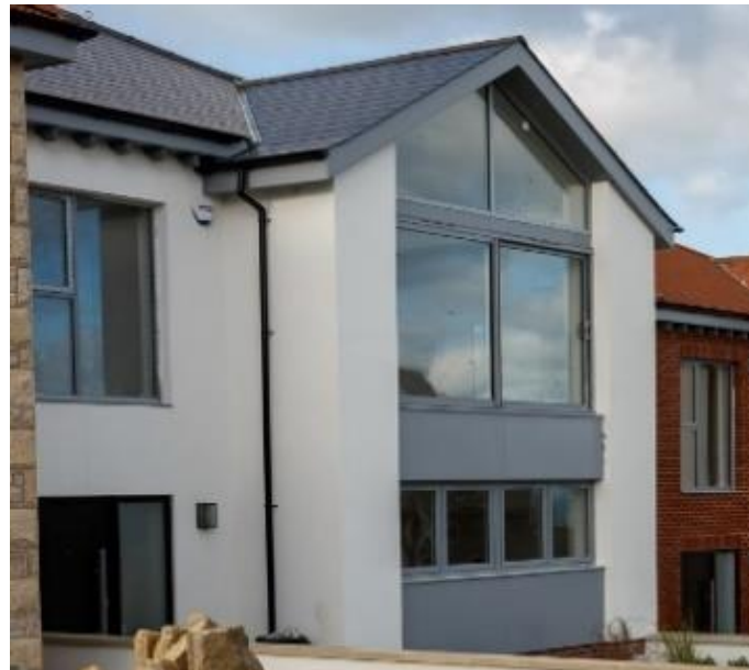
Fascias, soffits and guttering
