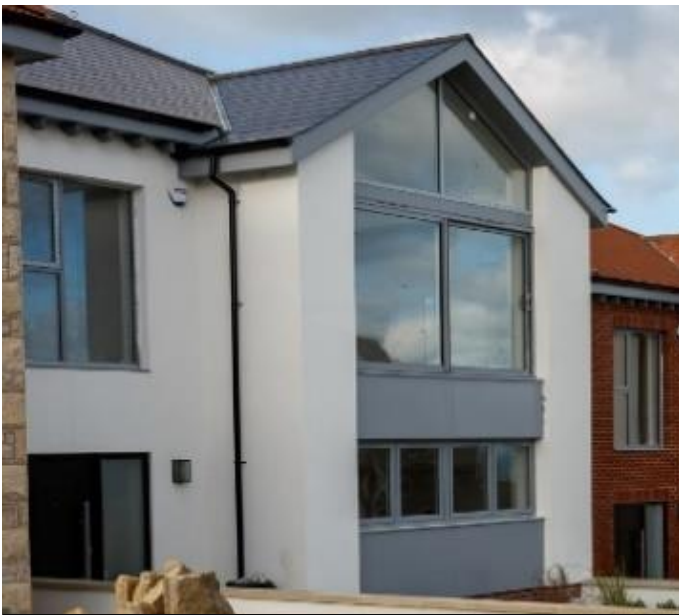
Fascias, soffits and guttering
