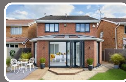
New Build Warm Rooms
