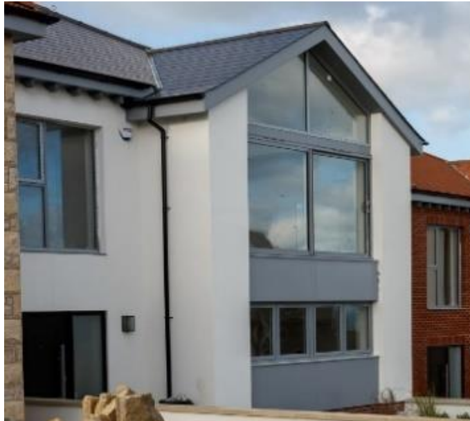
Fascias, soffits and guttering
