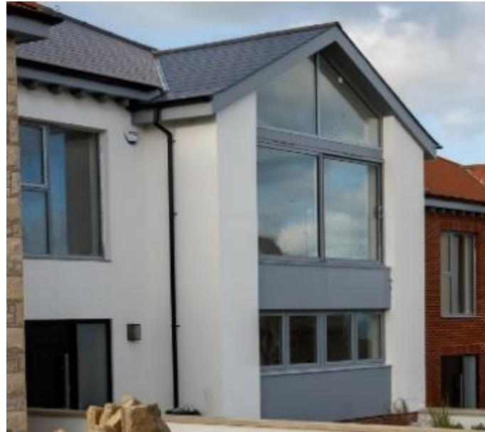
Fascias, soffits and guttering
