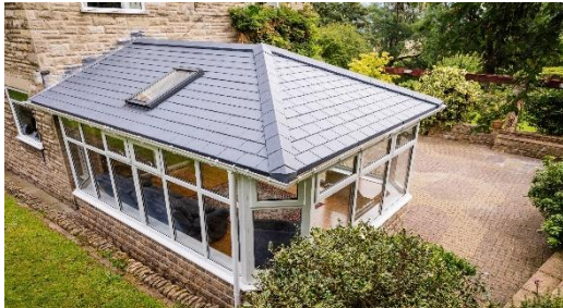
Conservatories and Equinox tiled roofs
