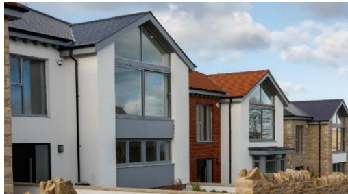
Fascias, soffits and guttering
