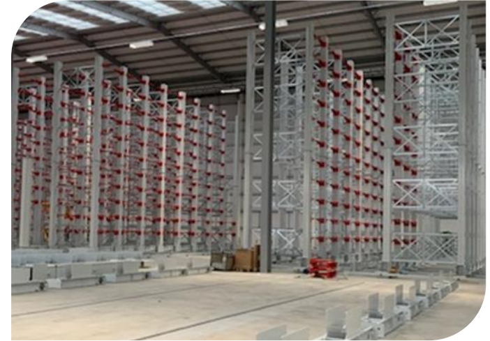
Mobile Racking Fit-out
