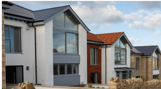
Fascias, soffits and gutters
