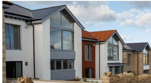
Fascias, soffits and gutters
