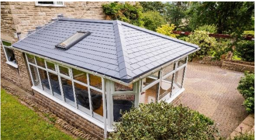
Conservatories and Equinox tiled roofs
