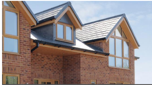
Fascias, soffits and guttering
