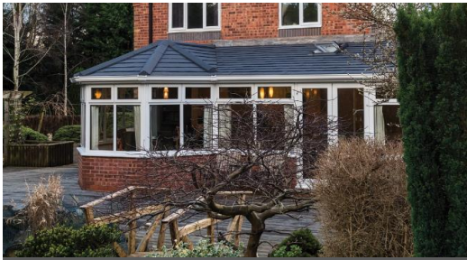
Conservatories and Equinox tiled roofs
