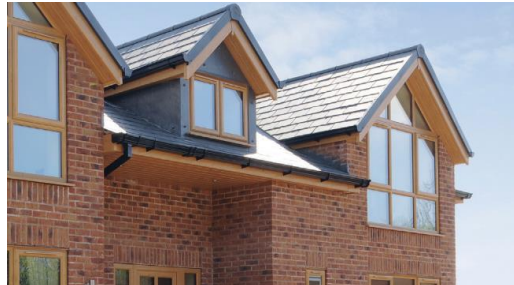
Fascias, soffits and guttering
