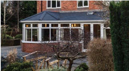
Conservatories and Equinox tiled roofs
