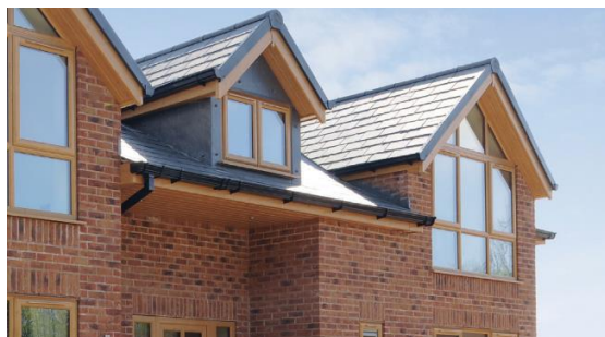
Fascias, soffits and gutters
